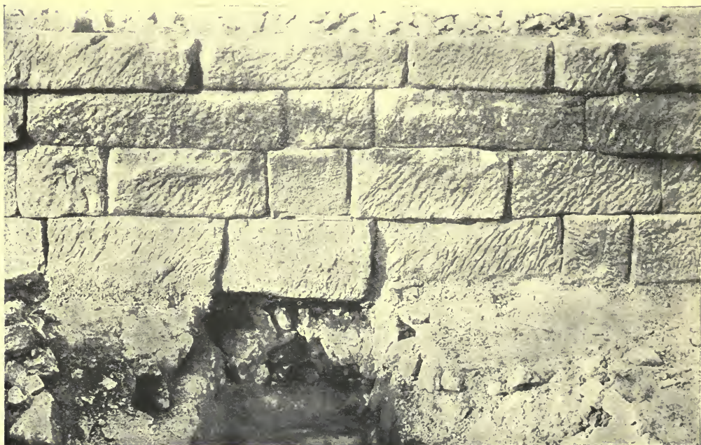
FIG. 28. EAST WALL OF PODIUM, COURSED MASONRY WITH CLAY AND RUBBLE FOUNDATIONS
